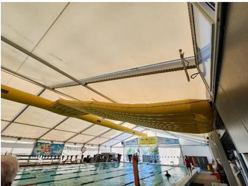
The pool shade structure has been supplied by "Karl Hocker Stahlbau GmbH, Germany" and has been constructed about 2002. The structure comprises aluminium portal frames, stainless steel bracing cables and mild steel components like base plates and some connection elements.
